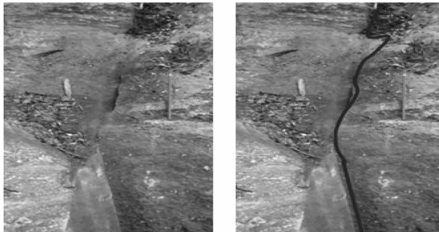
Figure 2c. ESE-WNW Fracture in the rock
