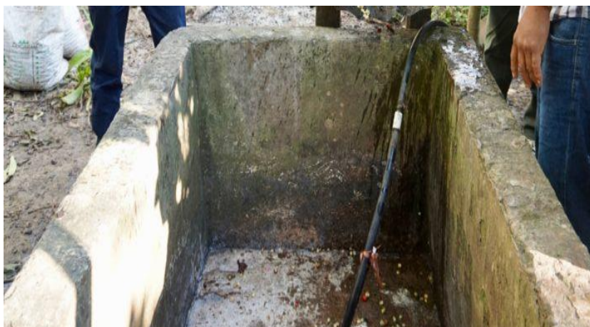
Figure I-6: Station de lavage
