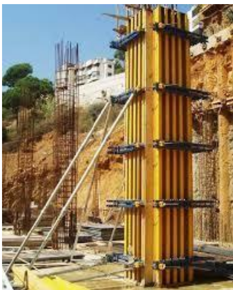
Figure 10: coffrage poteau métallique
