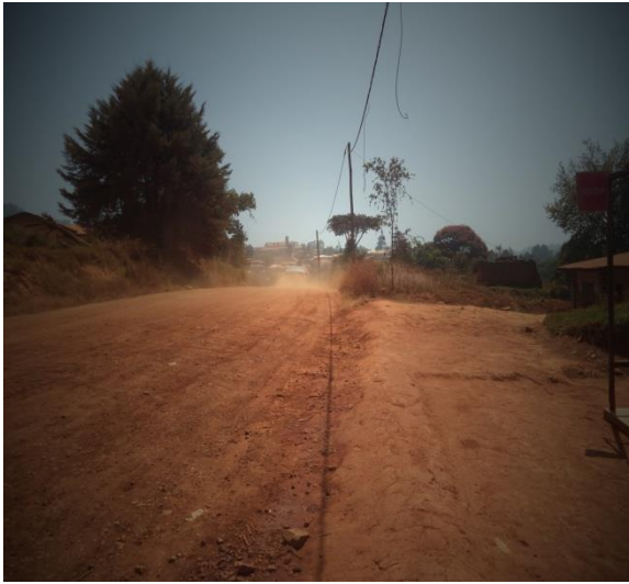
Picture 19: Poor state of the road
