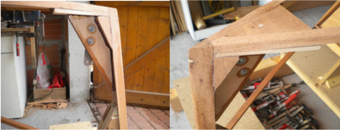
FIGURE 3.5 – Pose des renforts
