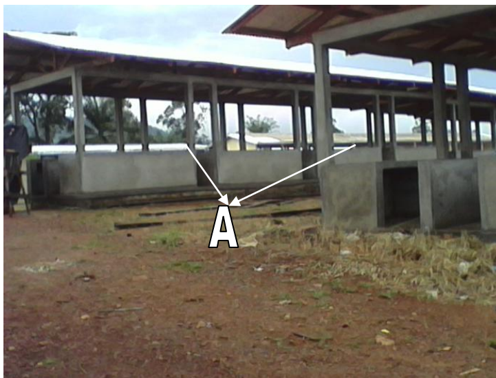
Photo 50: Mbon daily market under construction
