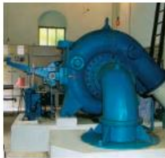
FIGURE 1.13 – Turbine Banki-Mitchell (cross-flow) [2]
