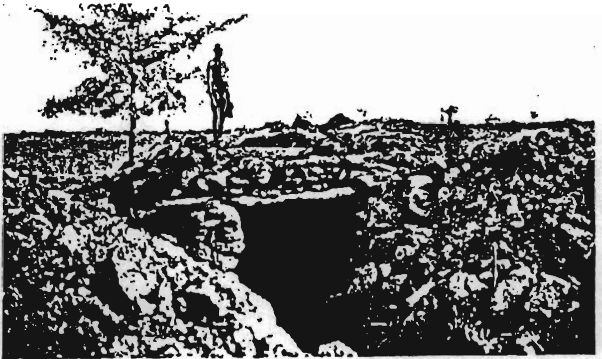
FIG. 4 - Iron furnace at Dédougou - subterranean self-draught type. Mill stalks, charcoal, and ore on platform at mouth of furnace.
