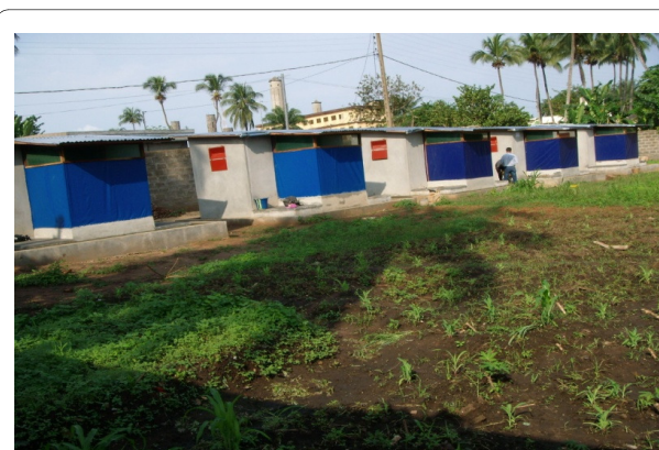
Figure 1 Experimental huts, Akron station. Courtesy CREC (September 2007).
