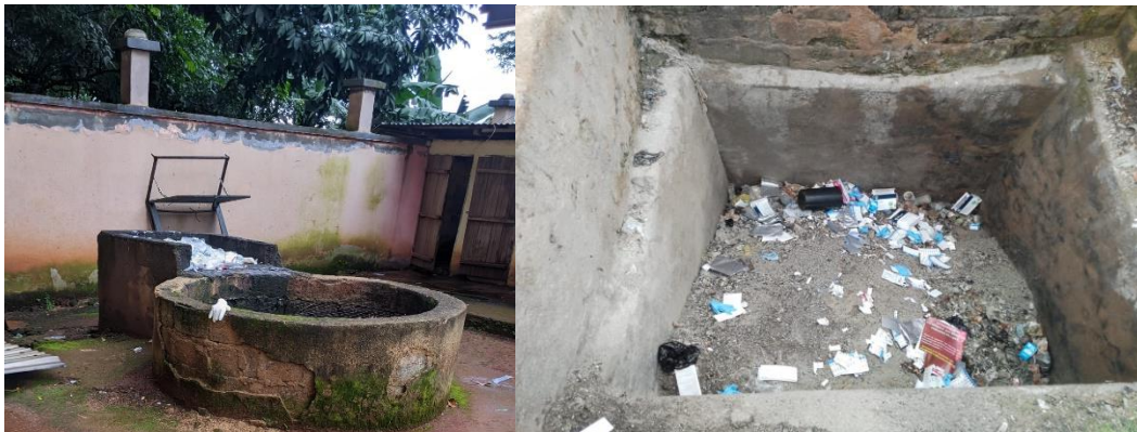
Figure 2: Open pit for liquid waste and open pit for solid waste dumping
