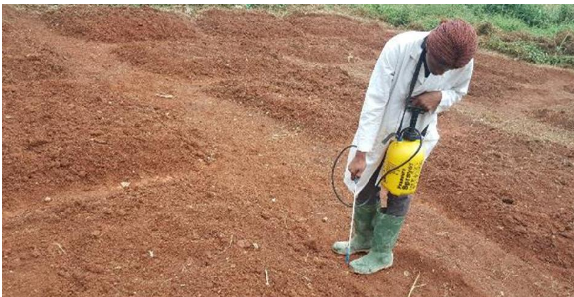
Fig. 14: Soil treatment. Insecticide (ACETAMIP surface sprayedsp)) was surface sprayed to prevent insect invasion.
