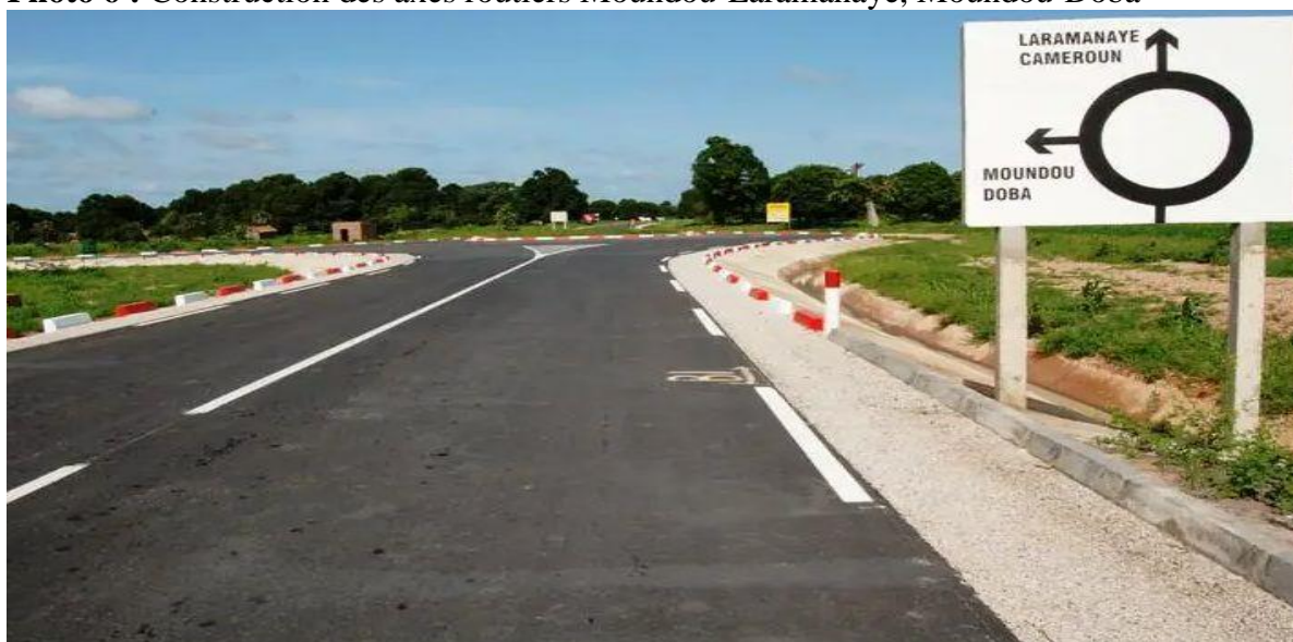
Photo 6 : Construction des axes routiers Moundou-Laramanaye, Moundou-Doba
