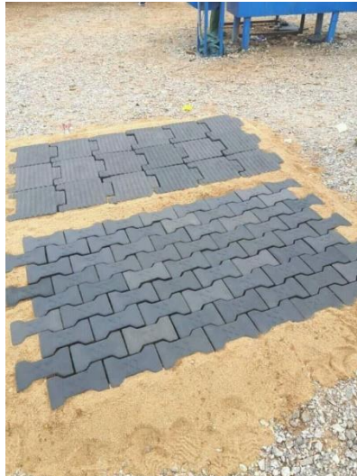
Photo 70: ... Transforming Waste: Pavements Made from Recycled Plastic by Coeur d'Afrique
