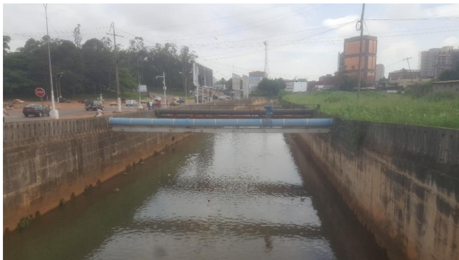
Photo 52 : Constructed work built to reduce flooding in the Central Town Source: Mbanam Valentine, 14 th September 2020
