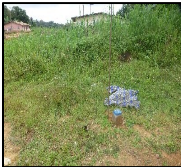
Photo 2d: Tombs demolished and demarcation for construction planted at Lobo
