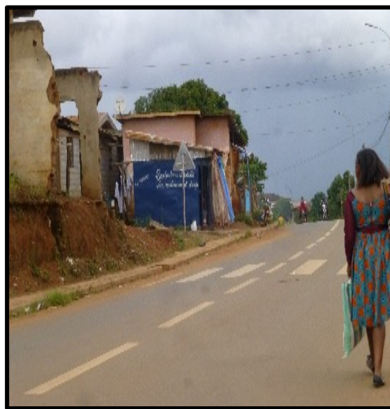
Photo 2b: Part of buildings destroyed at Mvog-Betsi
