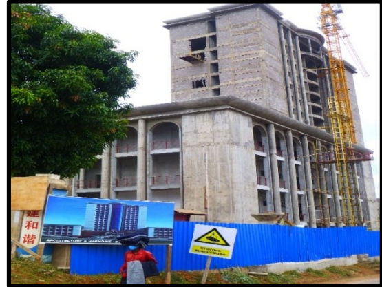
Construction site behind Palai de Justice
