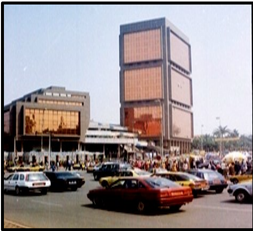
Ministerial building no 1
