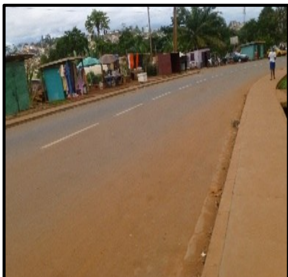
Photo 3c: Cross section of the Mvog-Betsi road.
