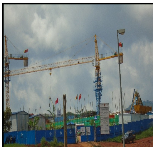
Construction site at Mballa 2
