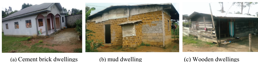
Figure 2. (a–c) Types of dwellings investigated in Ebolowa. (a) Cement brick dwellings; (b) mud dwelling; (c) Wooden dwellings.
