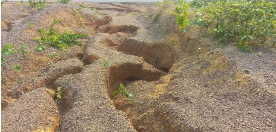
Photoboard 4a: gully erosion in Sangmelima
