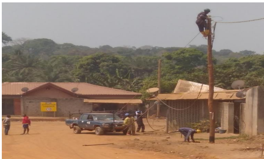
Photo 4: The ENEO agent on the field working on electric line extension
