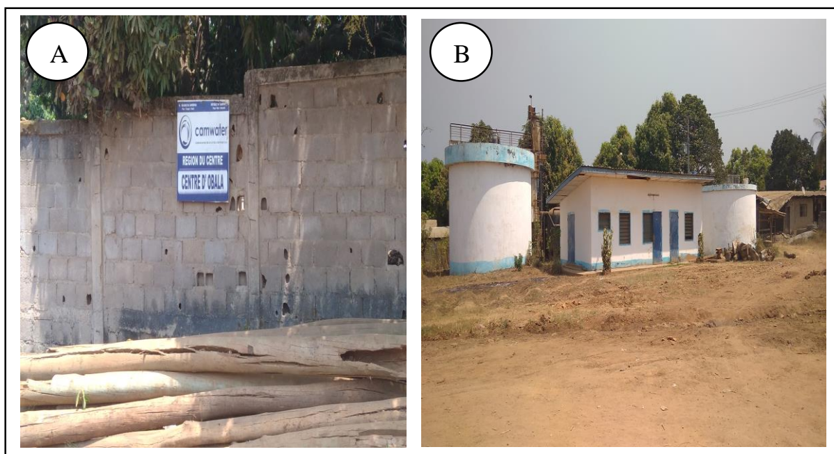
Plate 13: The CDE station which is now CAMWATER office in Obala
