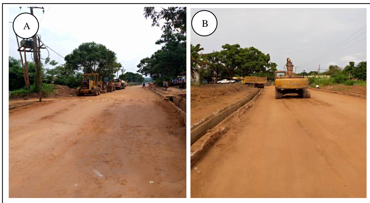
Plate 9: Road rehabilitation by the municipal Council
