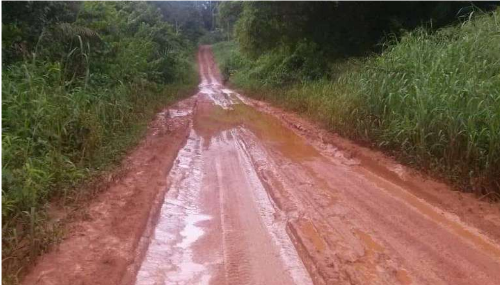
Picture 2: Ebolowa road linking kribi before tarring
