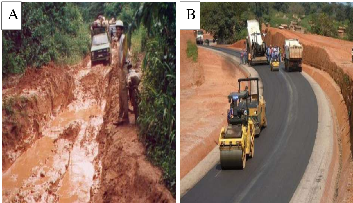
Plate 1: Ebolowa-Akom II road infrastructural changes
