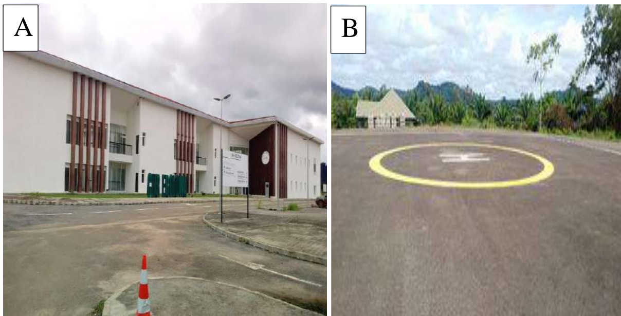
Plate 20 : The Regional Referral Hospital of Ebolowa
