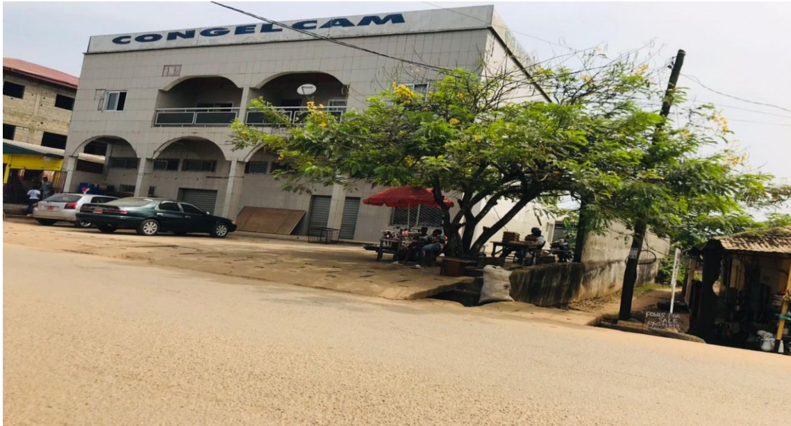
Photo 5: CONGELCAM building in Mamfe town
